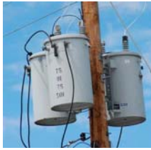
STO-50 is a 100% silicone formulated for use in liquid filled transformers.
